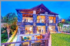
BALLITO BEACH HOUSE VILLA
